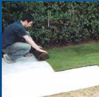
Directly under turf ensure that Stratacheck joins are butted and not overlapped.
