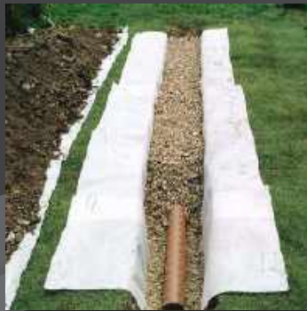
Land drain & Material storage
