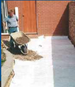
Domestic Patio under construction
