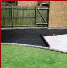
Under Domestic Patio Construction
