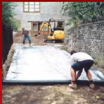
Under aggregate driveway
